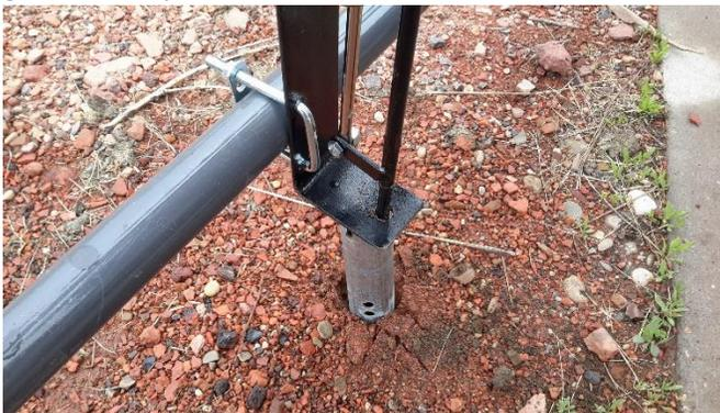
\* **Important Note:** If the gate is located on uneven ground, a wood post will need to be set to attach the pipe to. The pipe will then need to be attached to the post with lag bolts.
