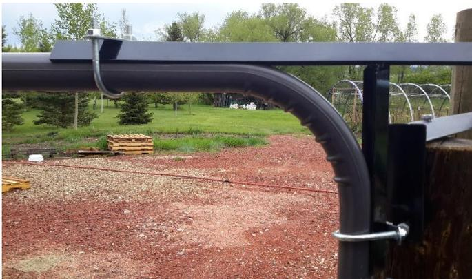
2. Attach “L” bracket to the top of gate hinge post using two of the lag bolts provided. First, install the lag bolt that screws into the top of the post, making sure that the front of the “L” bracket fits firmly against the side of the post, as shown in figure 2.
