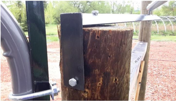
3. Install the spring, by first installing the provided eyebolt into one of the 3 pre-drilled holes on the end of the "L" bracket. Next attach the spring to the end of the "T" bracket and the eyebolt installed on the "L" bracket. Once the spring is in place, rotate the "L" bracket until the end of the gate comes in-line with the gate latch post, then install the last lag bolt as shown in figure 3.
