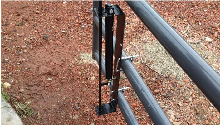
2. Fully open gate and mark the location where the time delay rod strikes the ground when pushed down. Do this for each direction the gate opens. Next drive the provided metal pipes into the ground at each location marked, so that the time delay rod will easily fit into the pipe when pushed down. The metal pipe should be positioned 1 inch below the bottom of the time delay bracket as shown in figure 6. In addition, the notch on the pipe should be facing towards the gate when opened.
